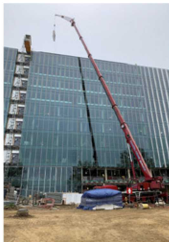
Crane at SSA
